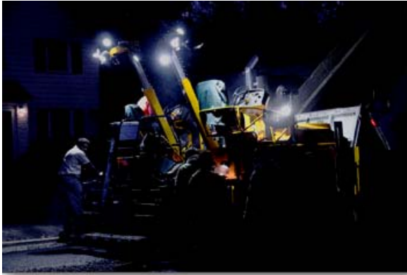
Night Team Paving. Bill Slack
